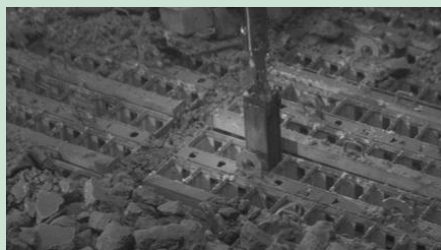
Spent fuel removal from Unit 3|TEPCO
