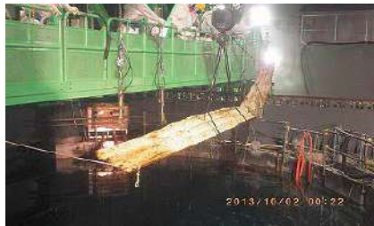
Retrieval of large rubble
